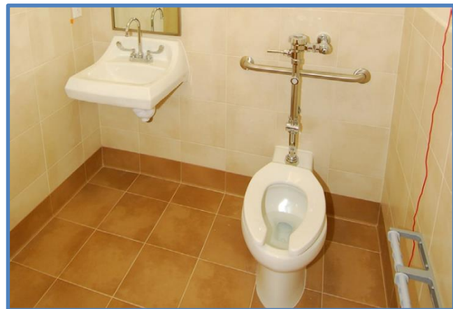
Figure 8: Typical bathroom with ADA handrail installed behind the toilet. (Multivista®)
