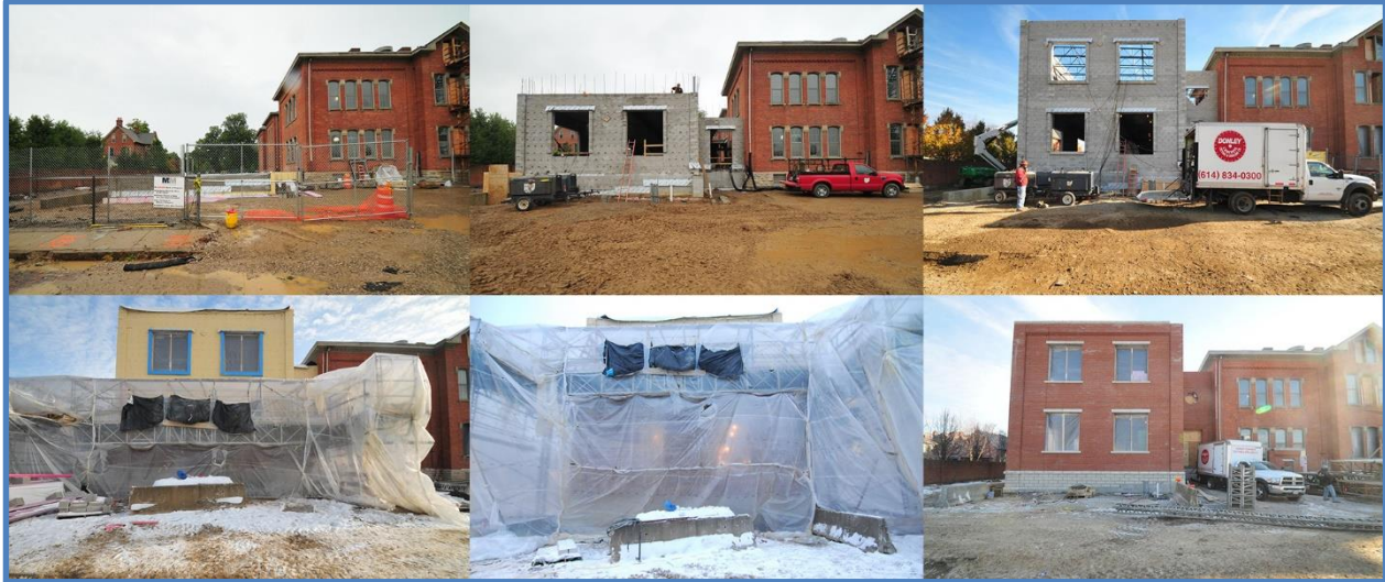
Figure 7: Example of exterior progression photos. (Multivista®)
